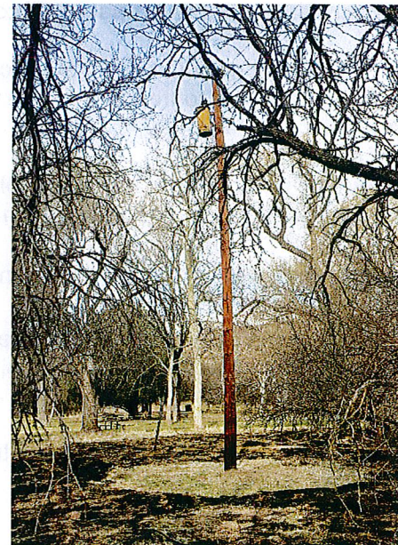
Example of Defensible Space Around Poles
