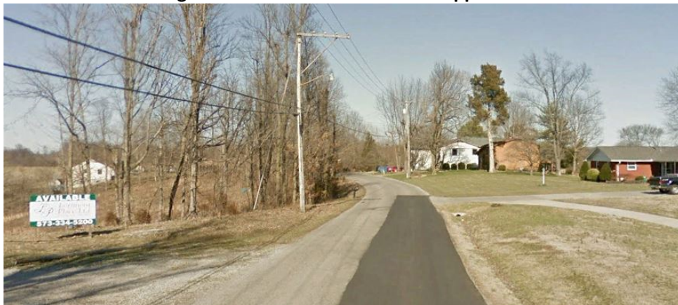
Figure 4: Northbound Curvature Approach
