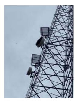
In order to replace the dish radome cover the dish has to be removed from the tower and lowered to the ground. Then a new cover can be installed. The dish then has to be raised back up the tower and re mounted. The dish was then aligned back into specifications towards the Franklin site.
