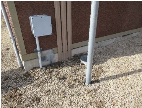
Ice Bridge Post #1 after Repair
