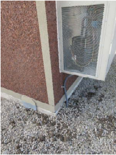
HVAC Ground after Repair
