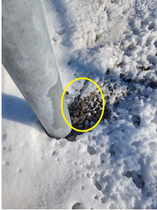
Ice Bridge Post #3 after Repair
