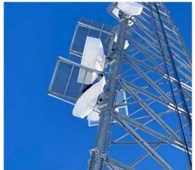
Motorola had a tower crew onsite on 2-21-25 and 3-6-25 to remove the last damaged 4ft dish and replace it with a new dish. The new dish required a new mount installed to properly align the dish.
