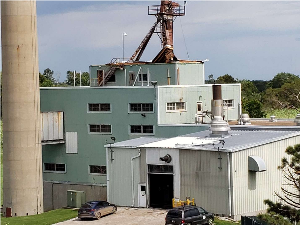
Power Plant Roof
