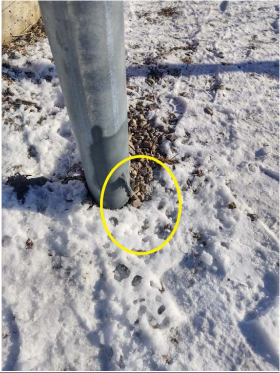
Ice Bridge Post #6 Ground Missing
