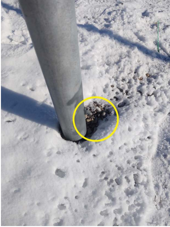
Ice Bridge Post #6 Ground Missing
