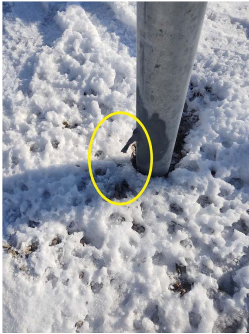
Ice Bridge Post #4 Ground Missing
