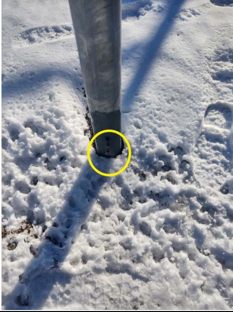
Ice Bridge Post #2 Ground Missing
