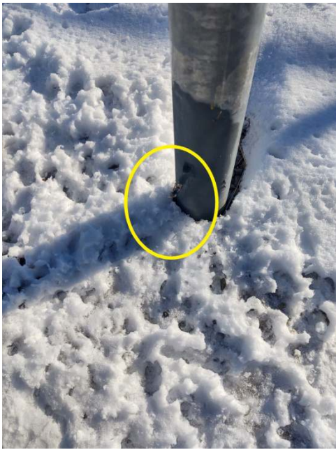
Ice Bridge Post #2 Ground Missing
