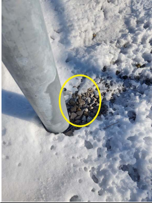
Ice Bridge Post #4 Ground Missing
