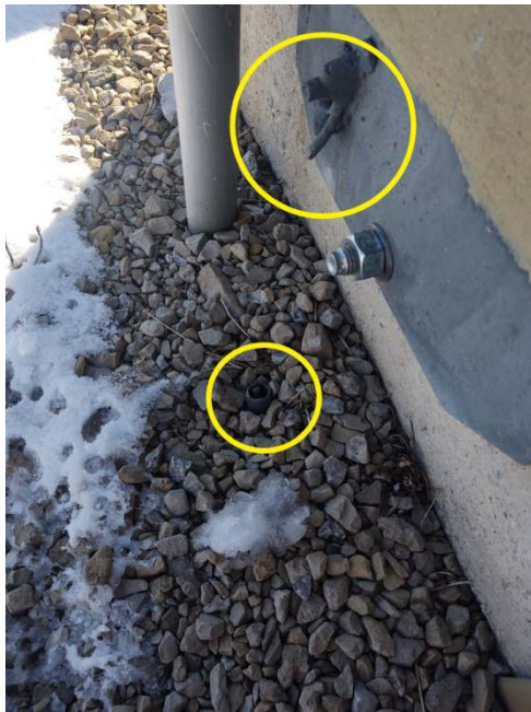
Shelter SE Corner Ground Missing
