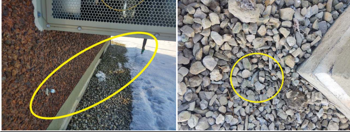
Shelter SE Corner Ground Missing
