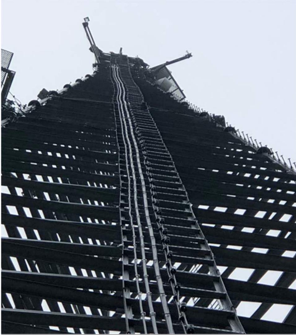
Microwave Link – Before and After Photos
