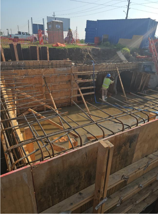
Figure 1: Rebar Inspection for junction box wall
