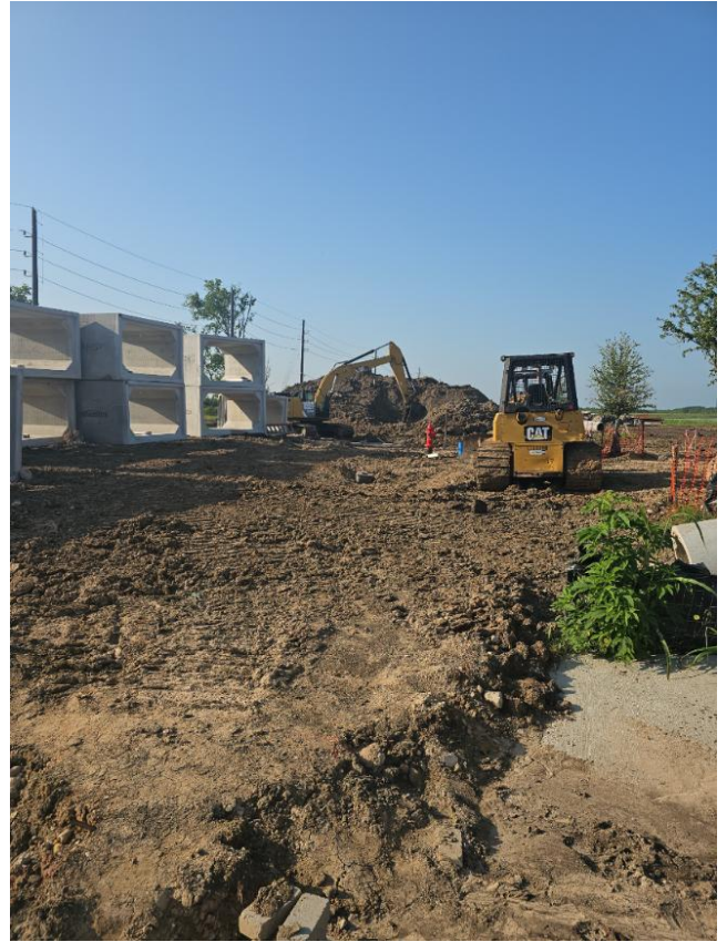
Figure 2: Preparation of site for installation of boxes
