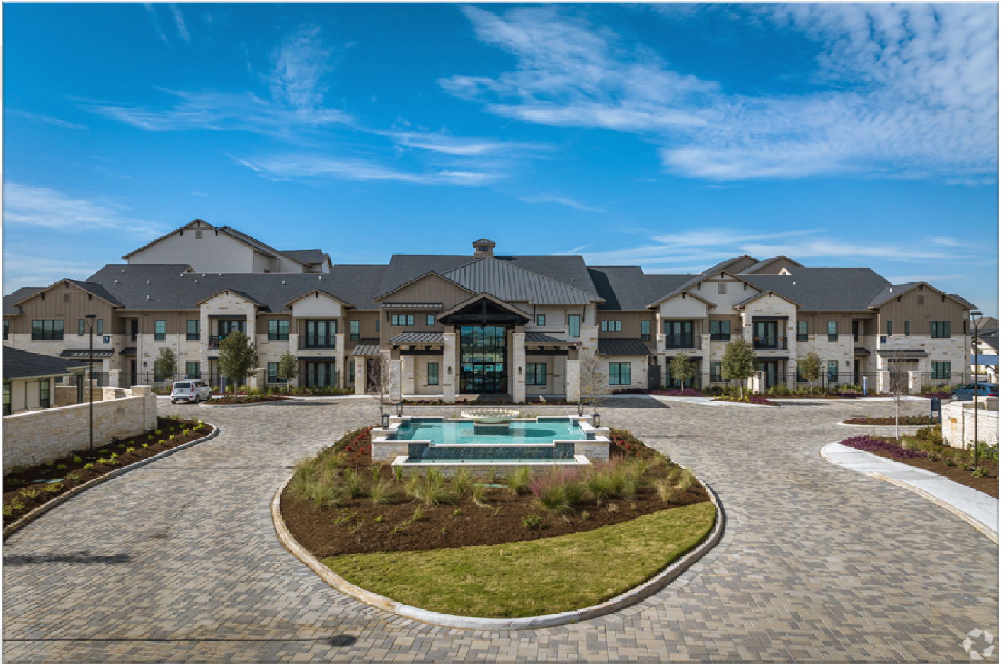
Typical Clubhouse Entry – Masonry with a mix of Cement Fiber Lap and Board & Batten Siding, Asphalt Shingle Roof
