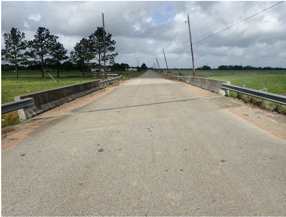
Figure G-3 View of survey Location "B"
