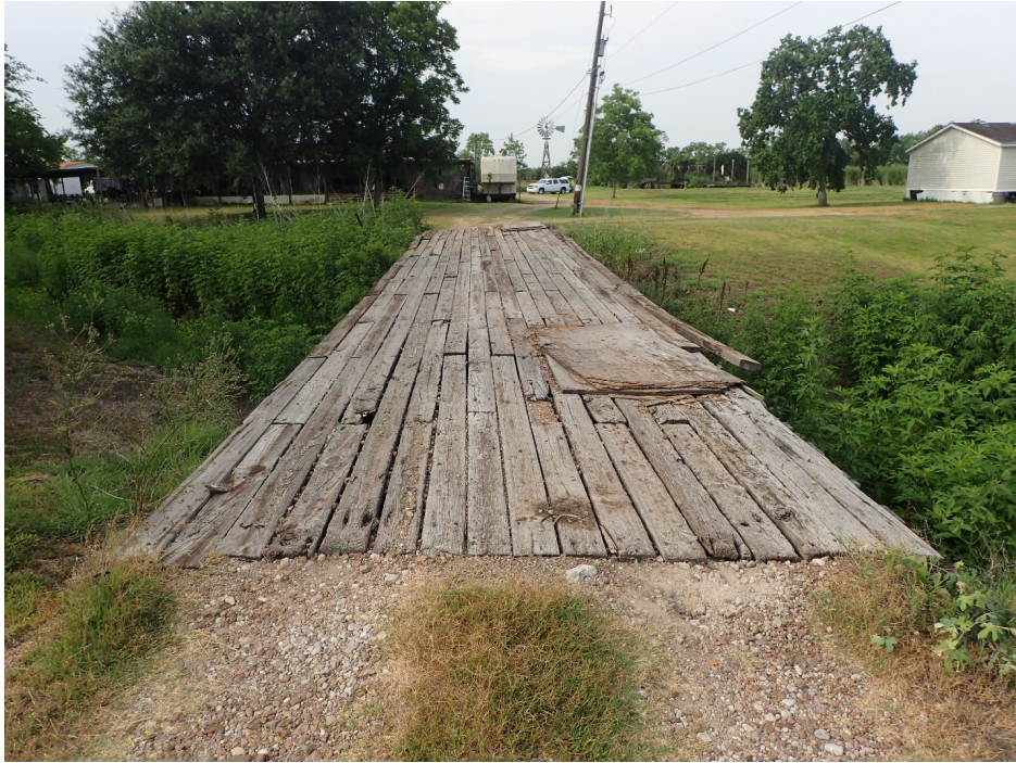
Figure G-13 View of survey location "H"
