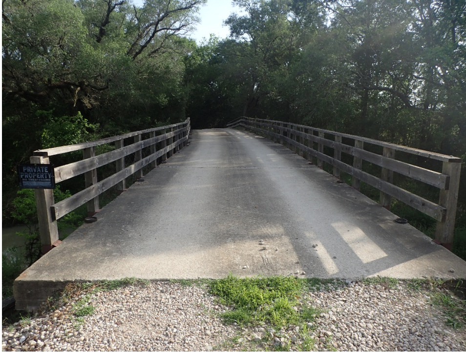
Figure G-7 View of survey location "D"
