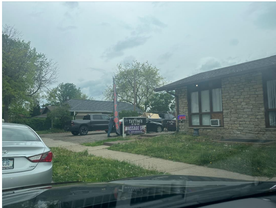
Looking northwest at primary building
