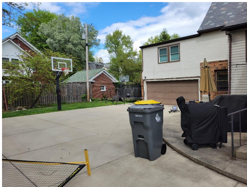
Photo 4: Existing Attached Garage Viewed from West
