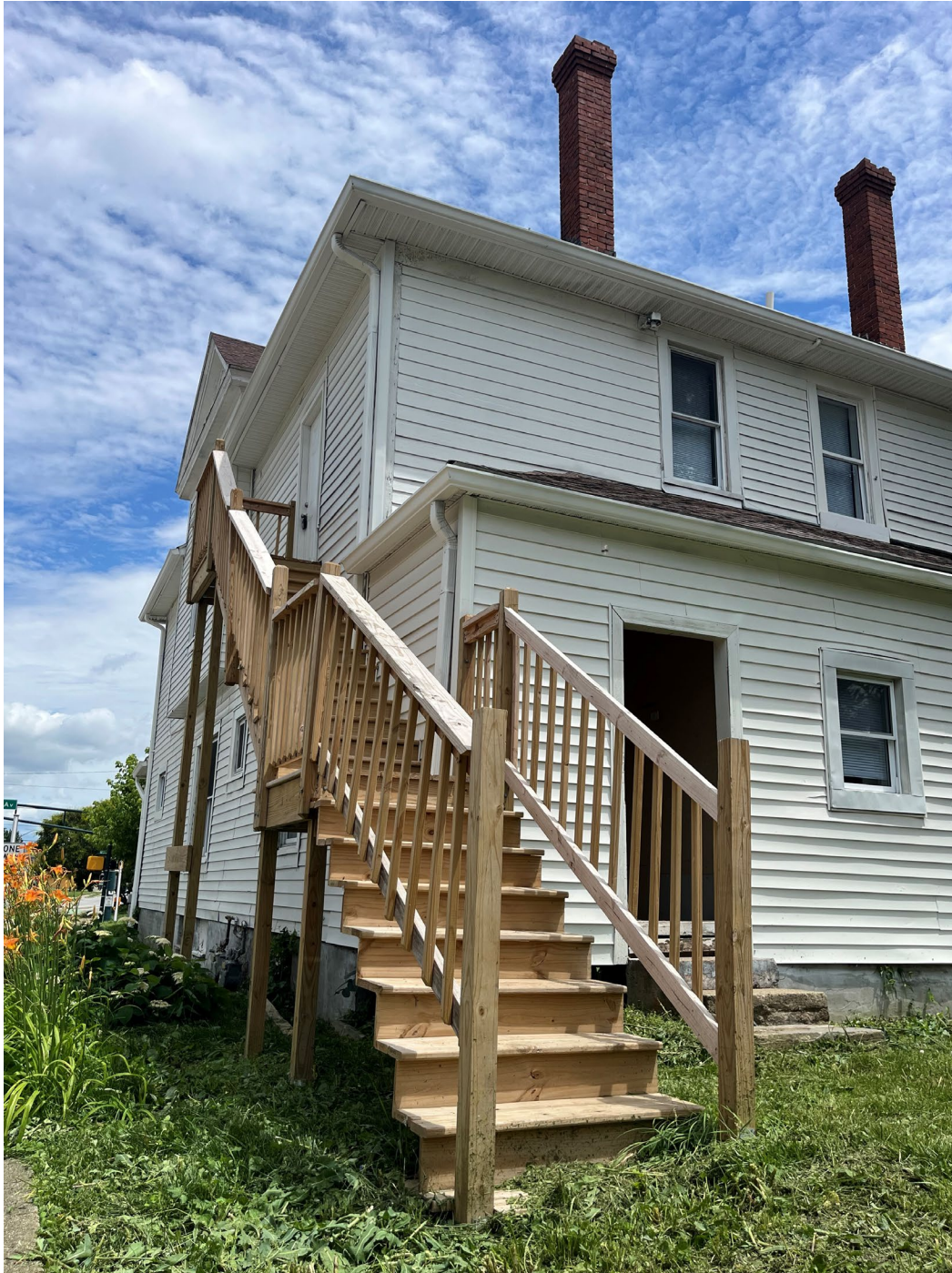
Photo 4: Another view of stairs from rear of property
