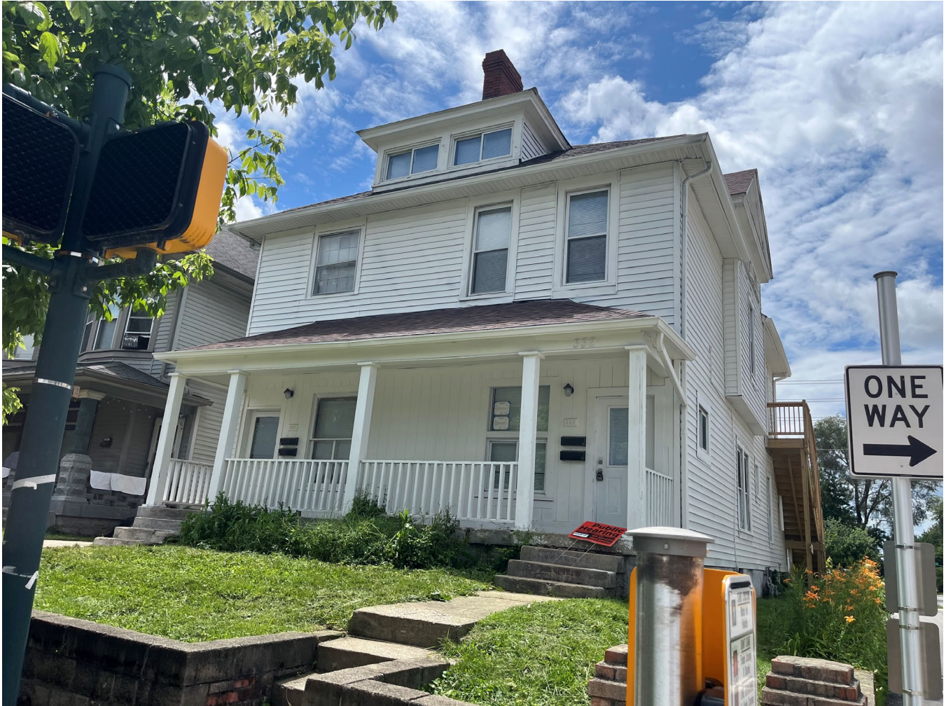
Photo 2: Close-up subject site from corner of Arsenal Avenue and New York Street
