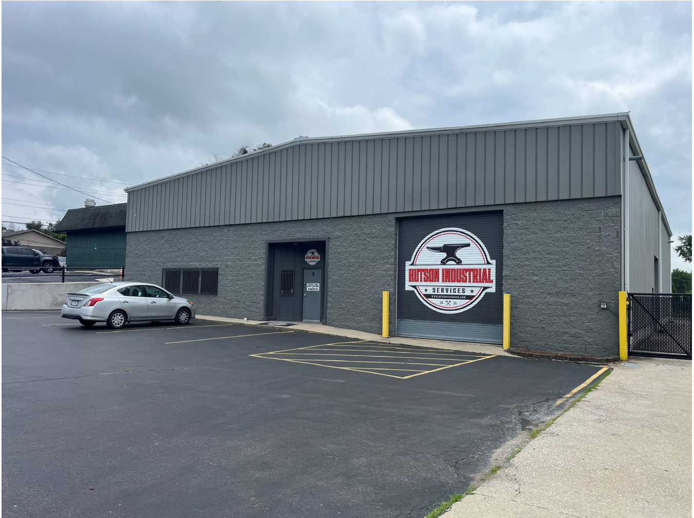
Photo 1: Subject site as seen from Epler Avenue
