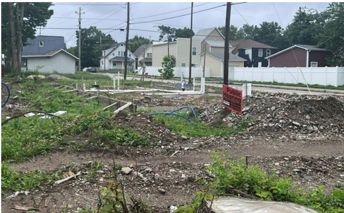
Looking Southeast towards the alley
