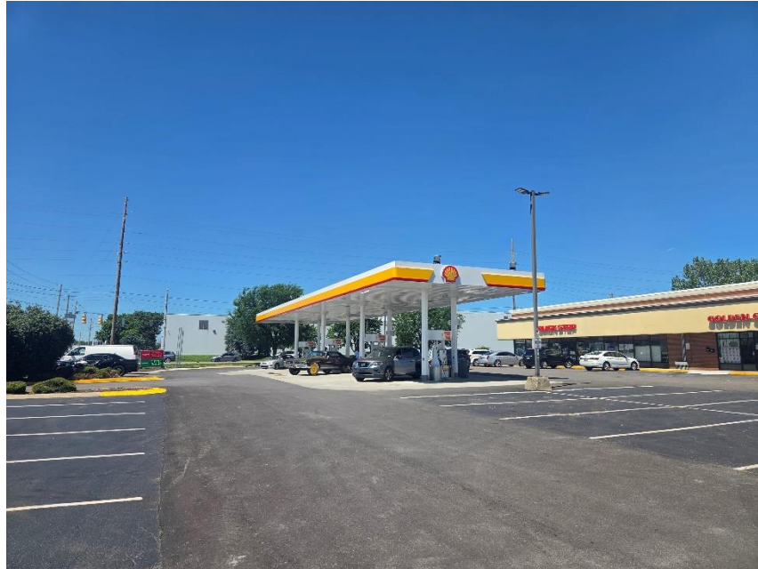
Photo 1: Extended Canopy Viewed from South
