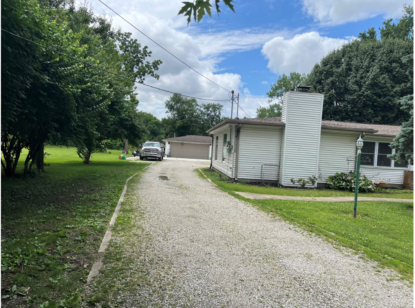
Photo 3: Property as seen from the driveway
