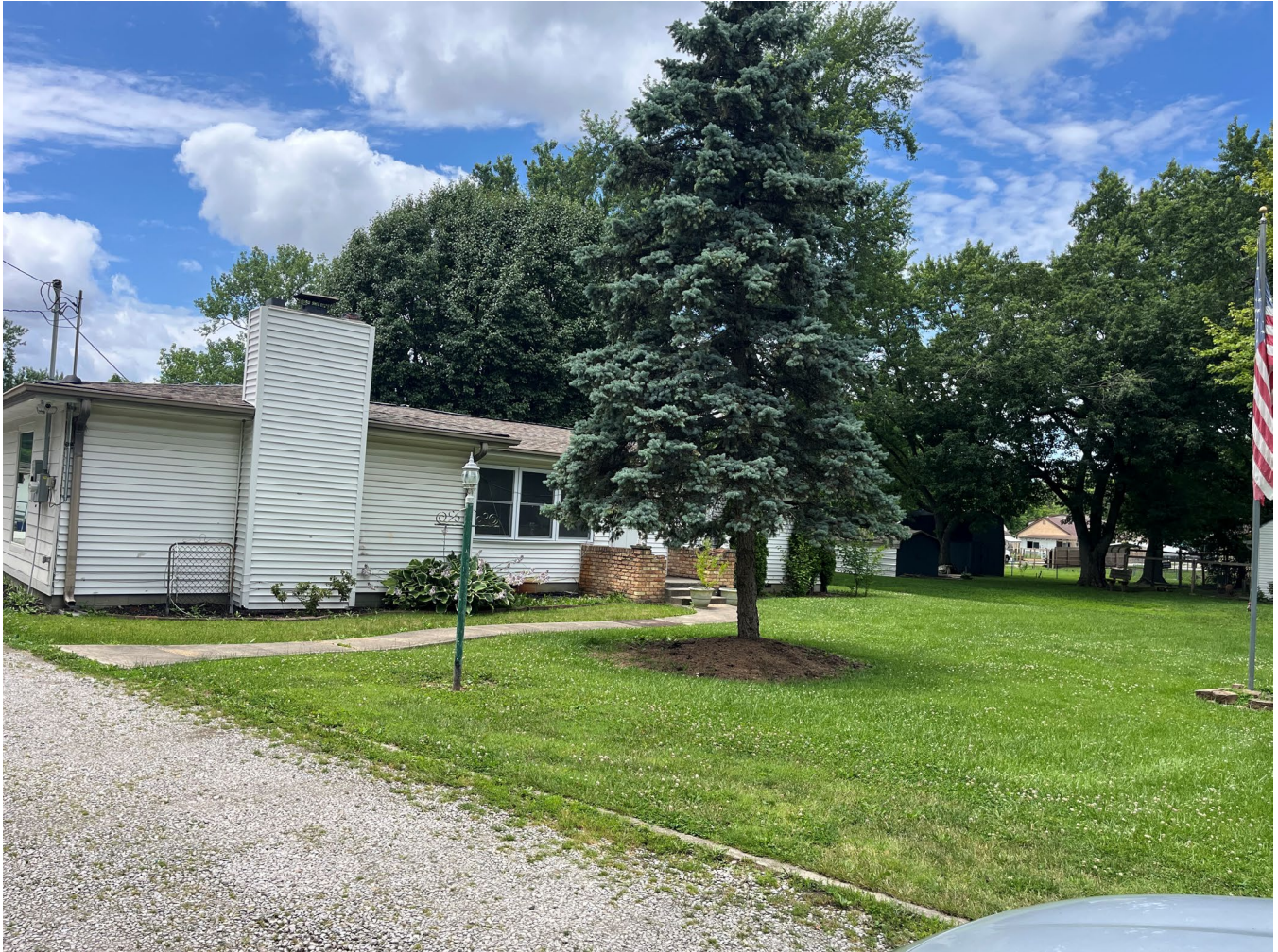
Photo 4: View of the front of the property
