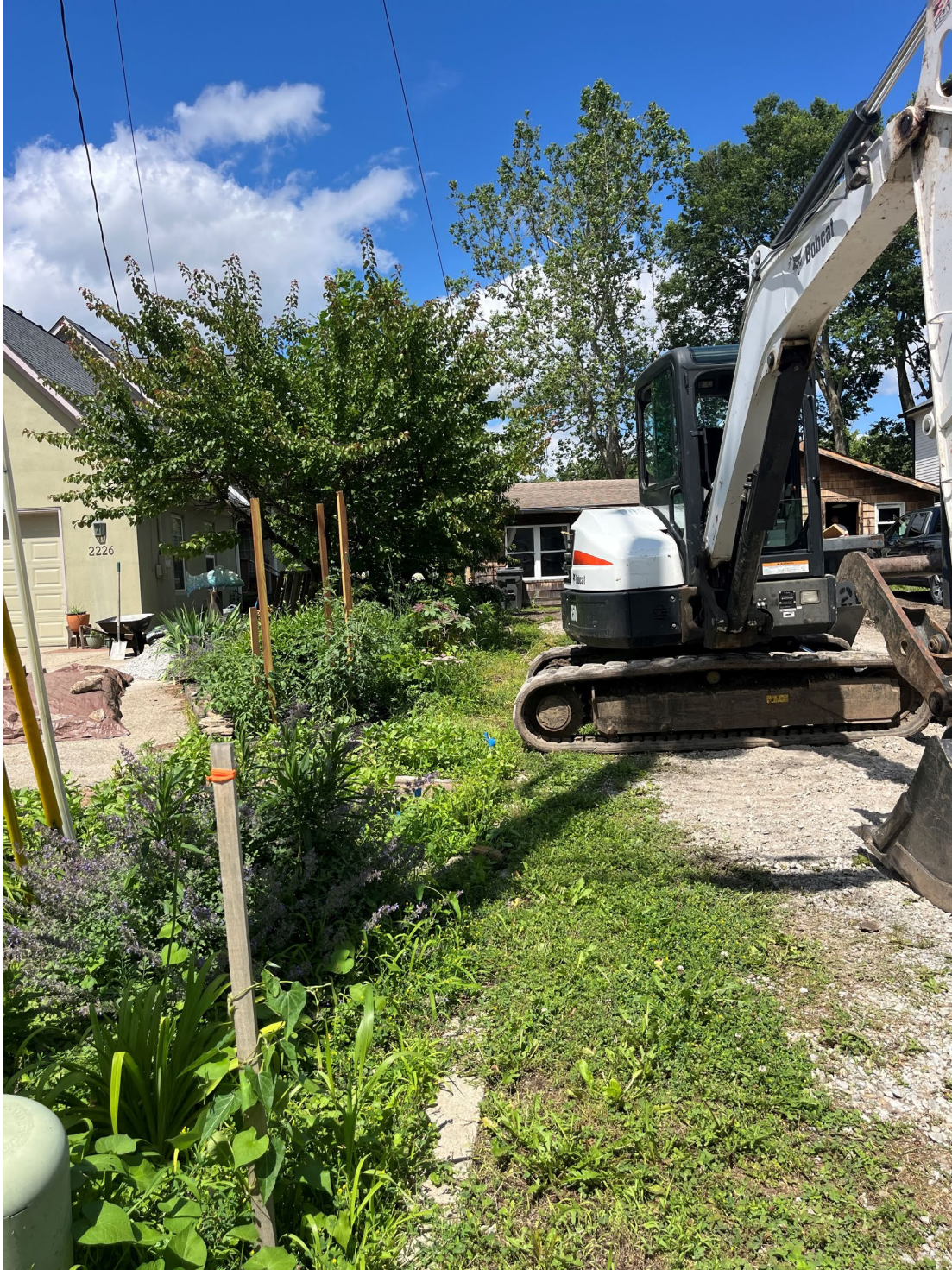
Photo 3: View of western side of property with stake showing property line
