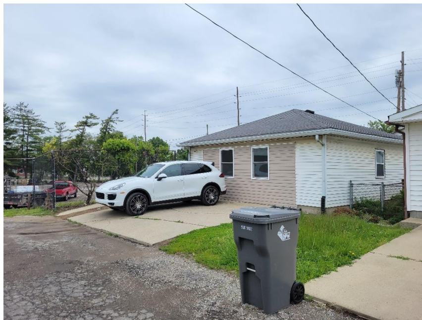
Photo 2: 2335 Morris Viewed from Southeast
