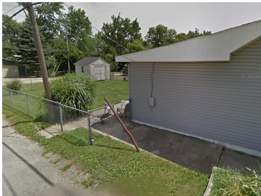
Photo 4: 1211 Tremont Viewed from North (July 2011)
