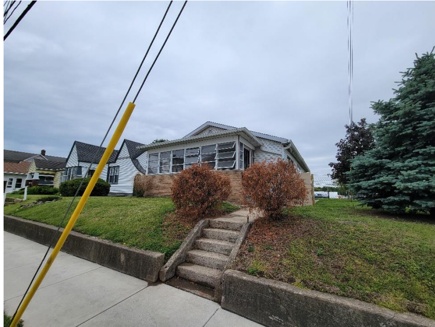
Photo 1: 2335 Morris Viewed from North
