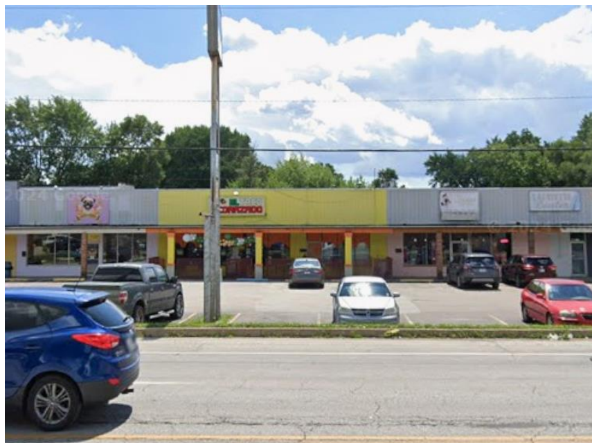
Photo 4: Subject Site Viewed from East (July 2024)
