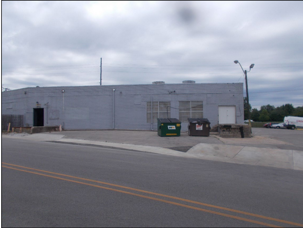
Looking north across 34 th Street the site.
