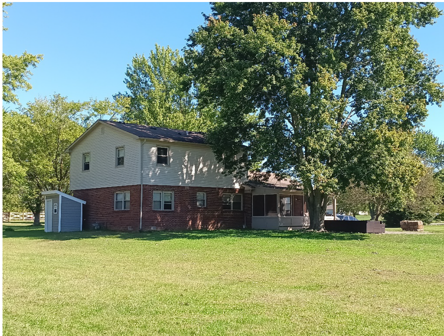
Exhibit 6: The back of the primary structure at 9621 E 96 th Street.
