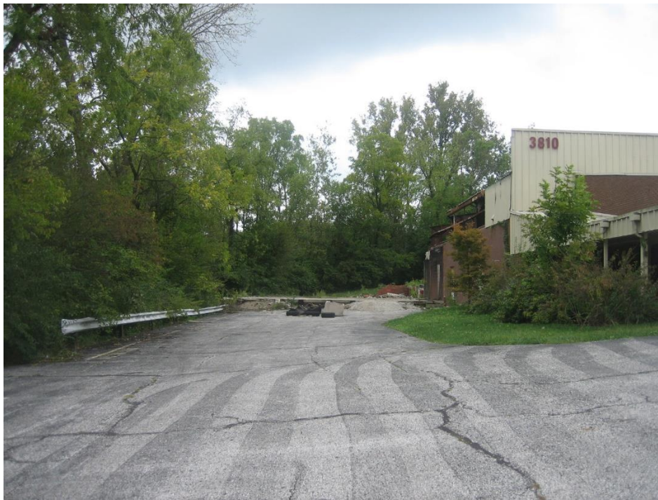
Subject site proposed expansion area, looking north
