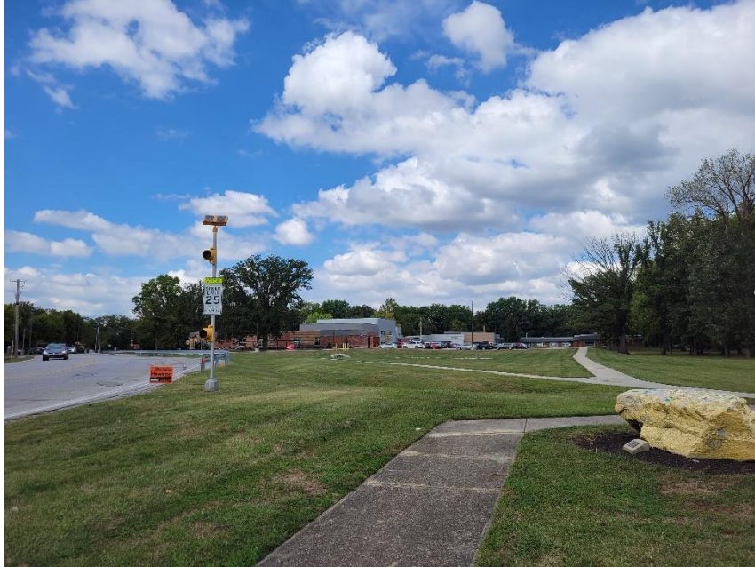
Photo 5: Subject School Viewed from South
