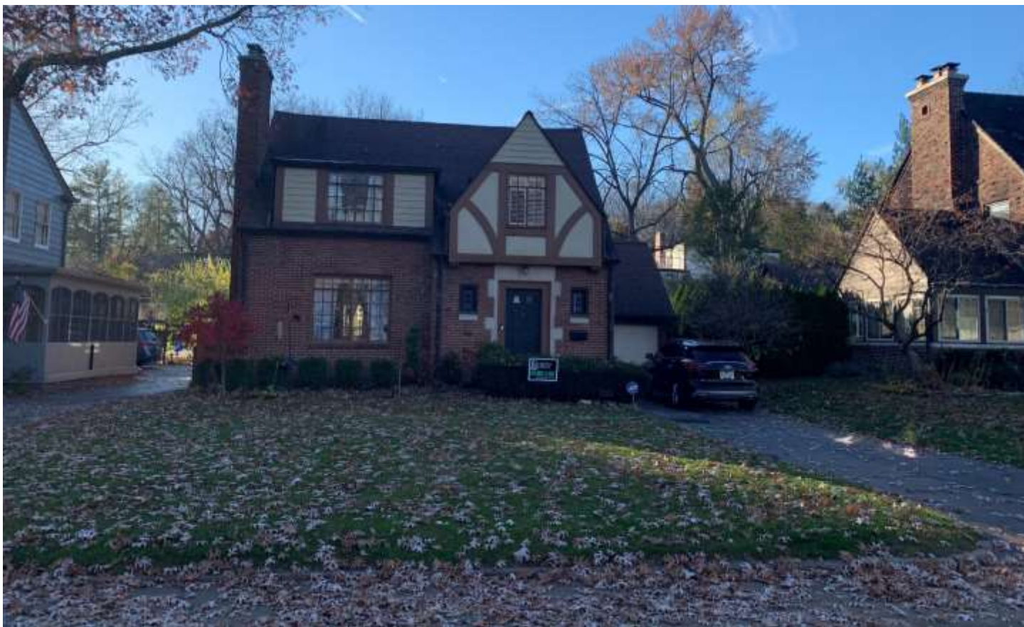
Photo of the Subject Property: 7036 Warwick Road
