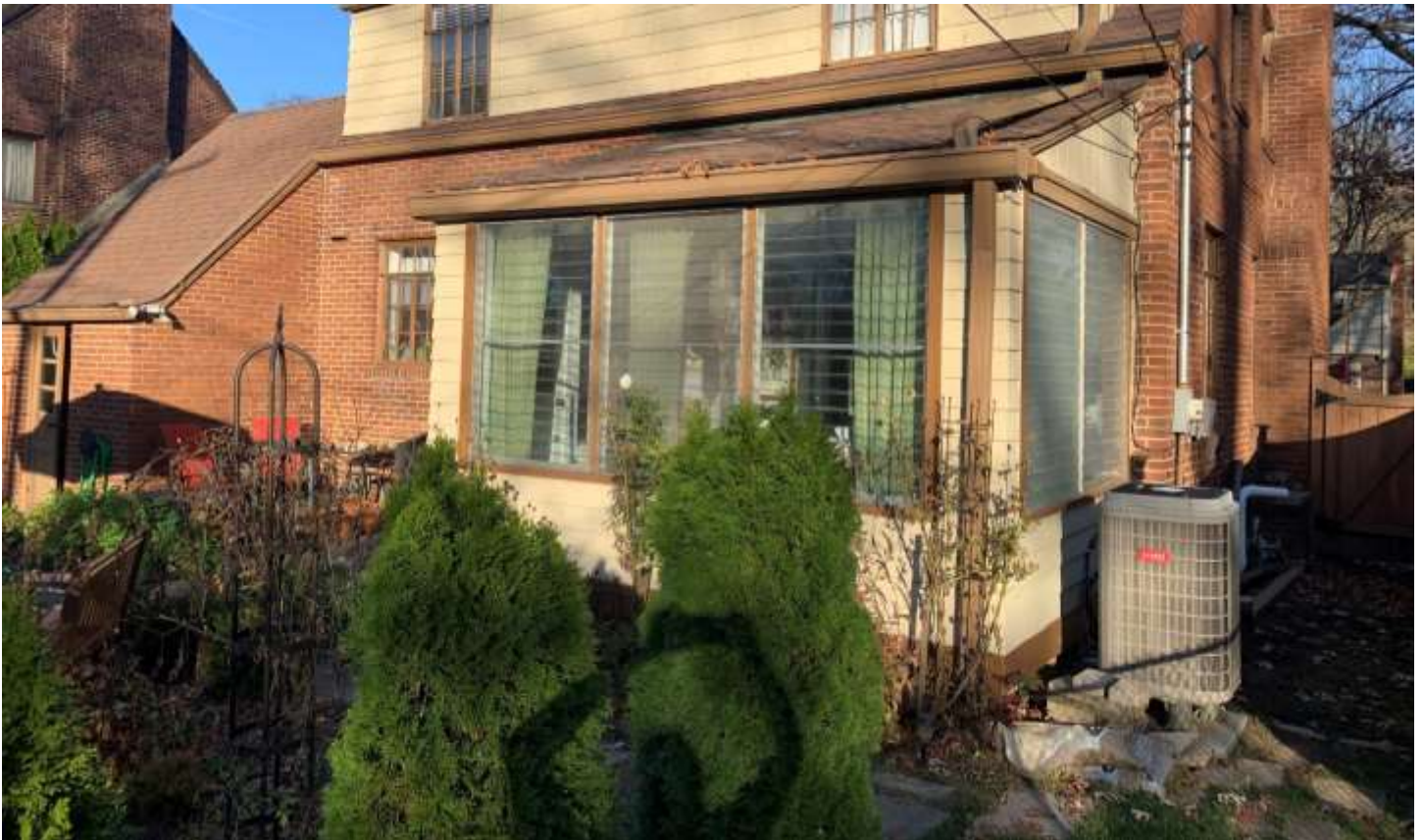
Photo of the location of the house additon to replace the sunroom.
