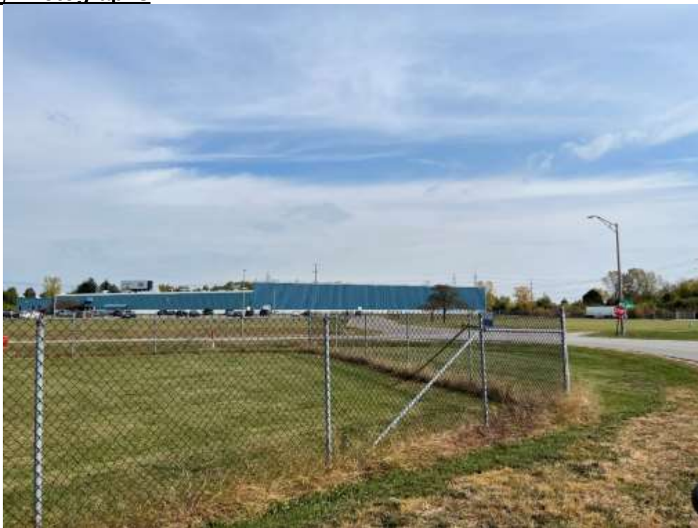
Photo of industrial property to the northeast.
