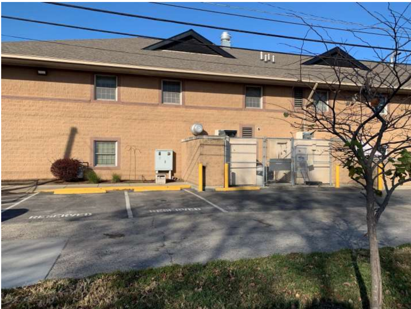
Photo of the additction treatment center north of the alley.
