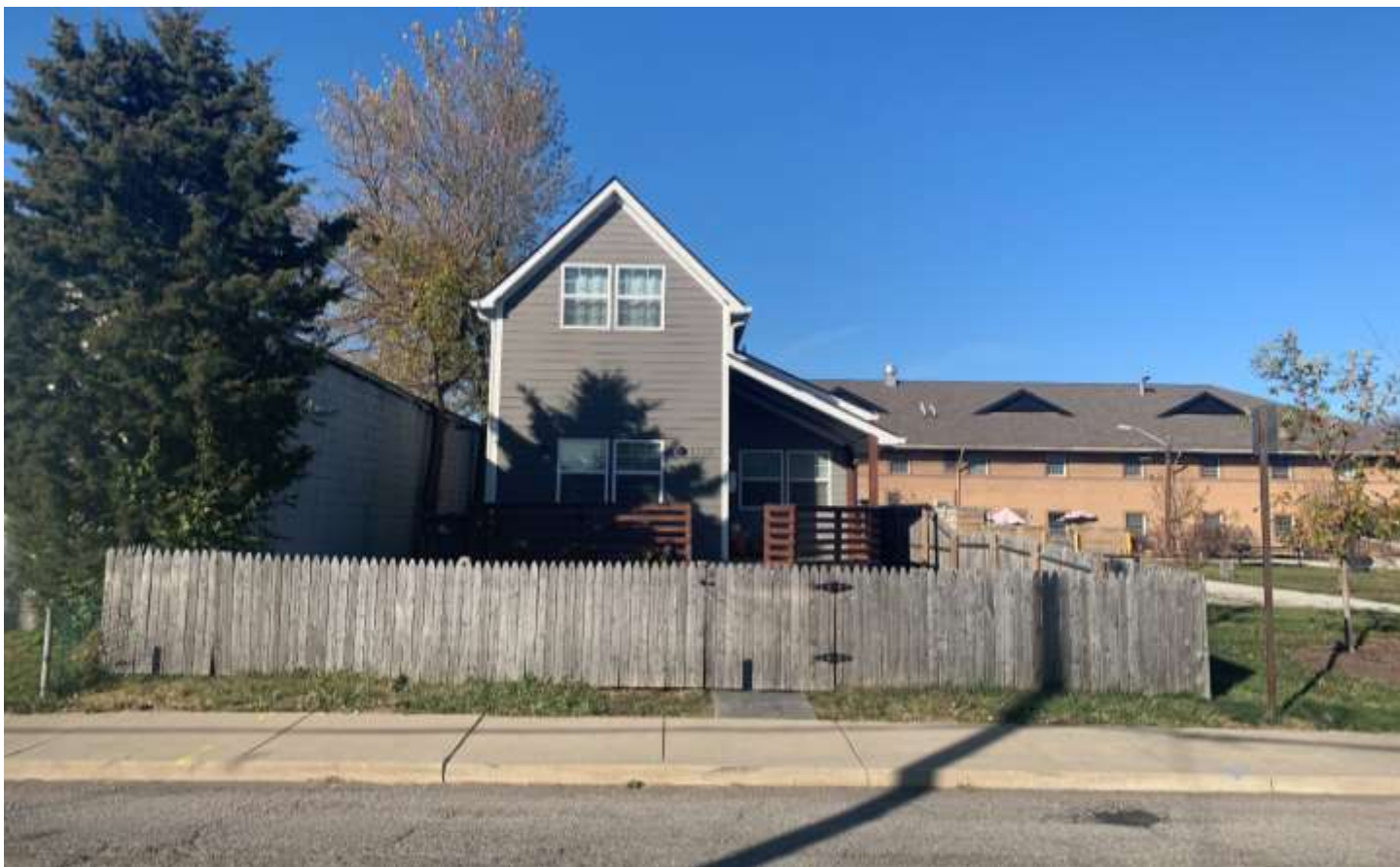
Photo of the Subject Property: 1110 Bates Street
