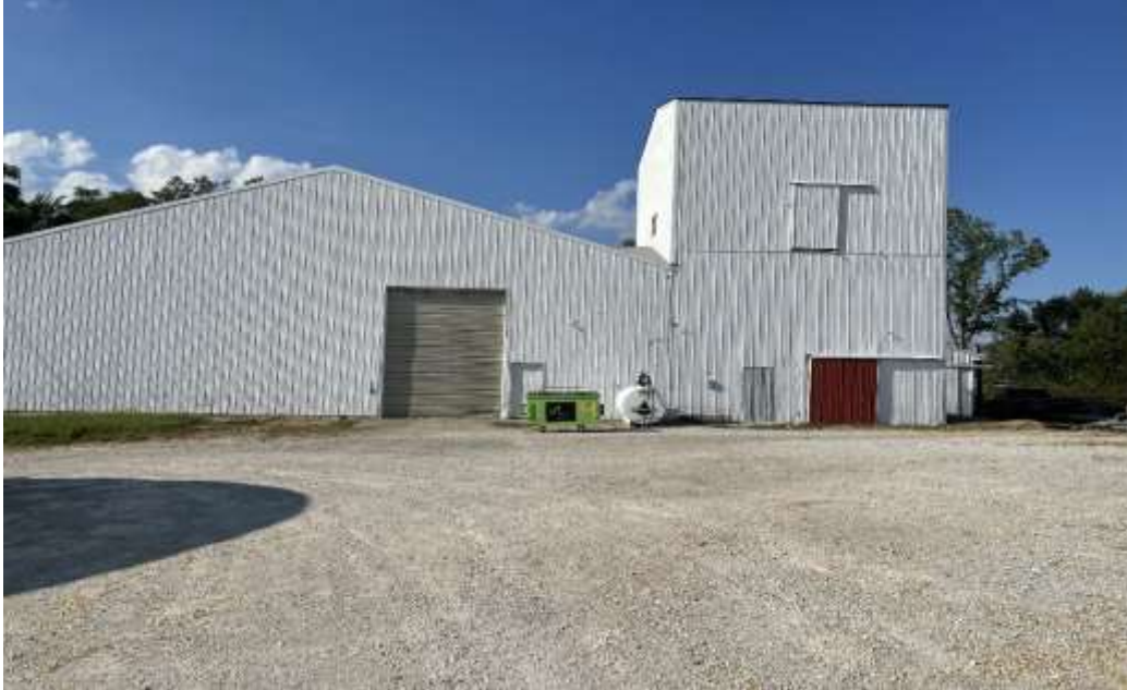
Photo Five: Primary Building For Assembly, Looking North
