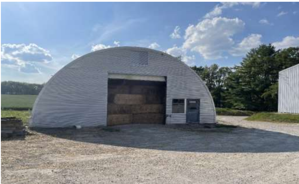
Photo Six: Storage Building, Facing West
