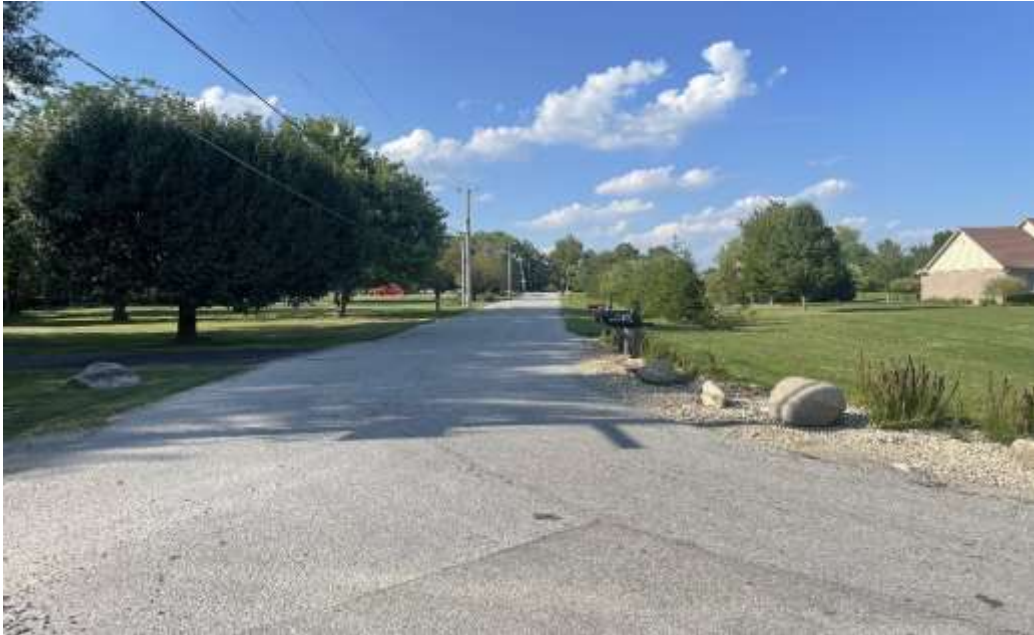
Photo One: Looking North Along Maze Road
