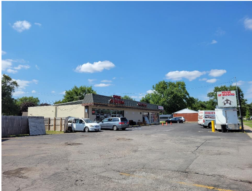
Photo 6: Adjacent Property to North
