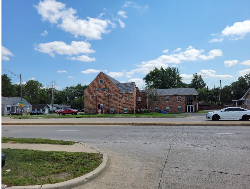
Photo 9: Adjacent Property to South
