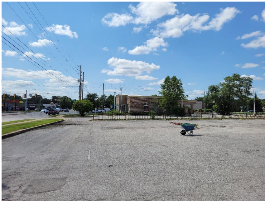
Photo 6: Existing Outlot on Southwestern Section of Site
