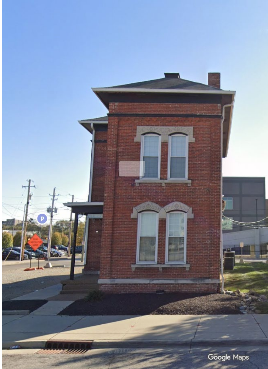
Photo 6: A recent image of the front of the subject site
