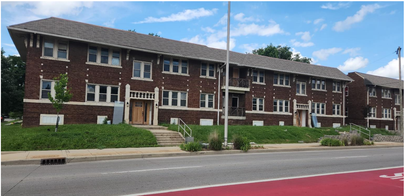
Subject site, 534 East 38 th Street, proposed fencing. Looking northeast.
