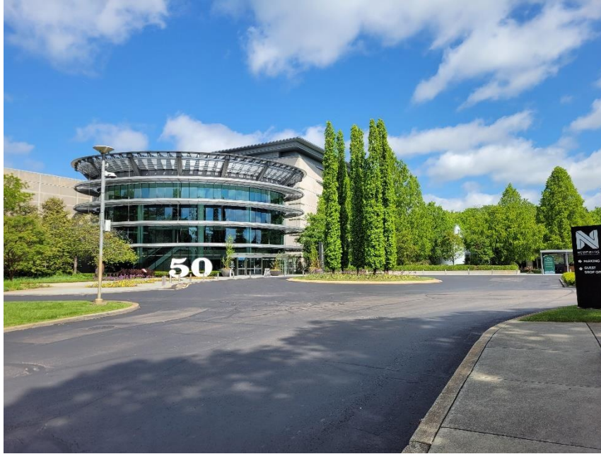
Photo 1: Primary Building Viewed from South
