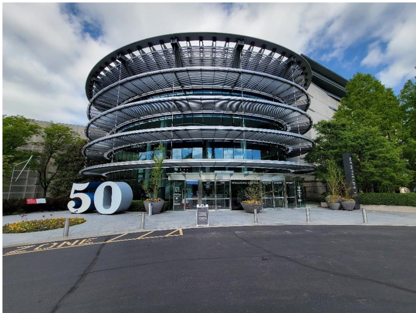
Photo 2: S1 Sign Location Viewed from West
