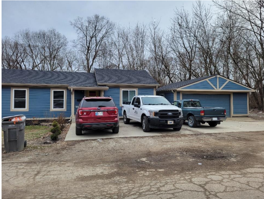
Photo 1: Subject Residence Viewed from North
