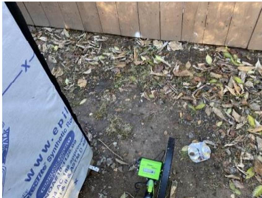
Photo 8: Separation Between Unpermitted Garage and Fence to East (November 2025)
