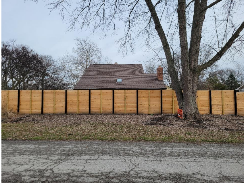
Photo 1: Fence from Front Yard (West)
