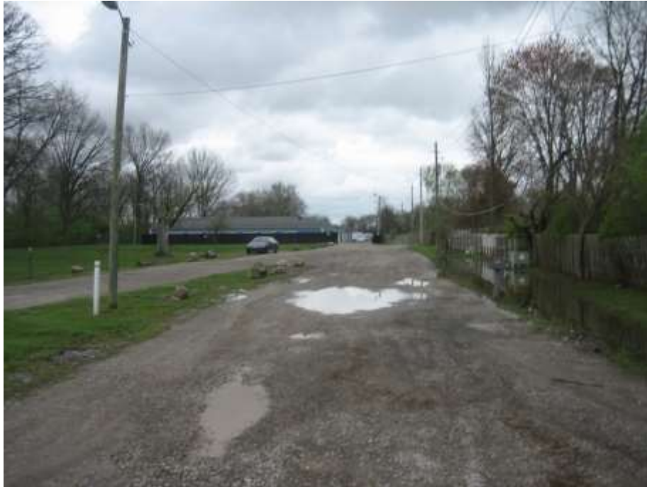
Subject site driveway from Morris Street, looking south
