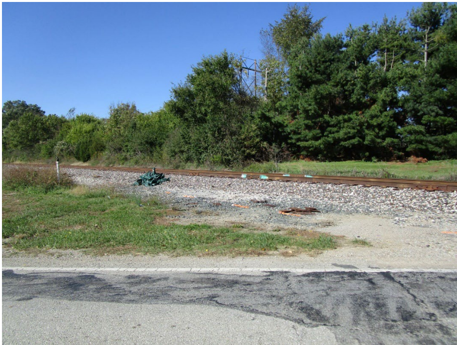
View looking north across East Edgewood Avenue
