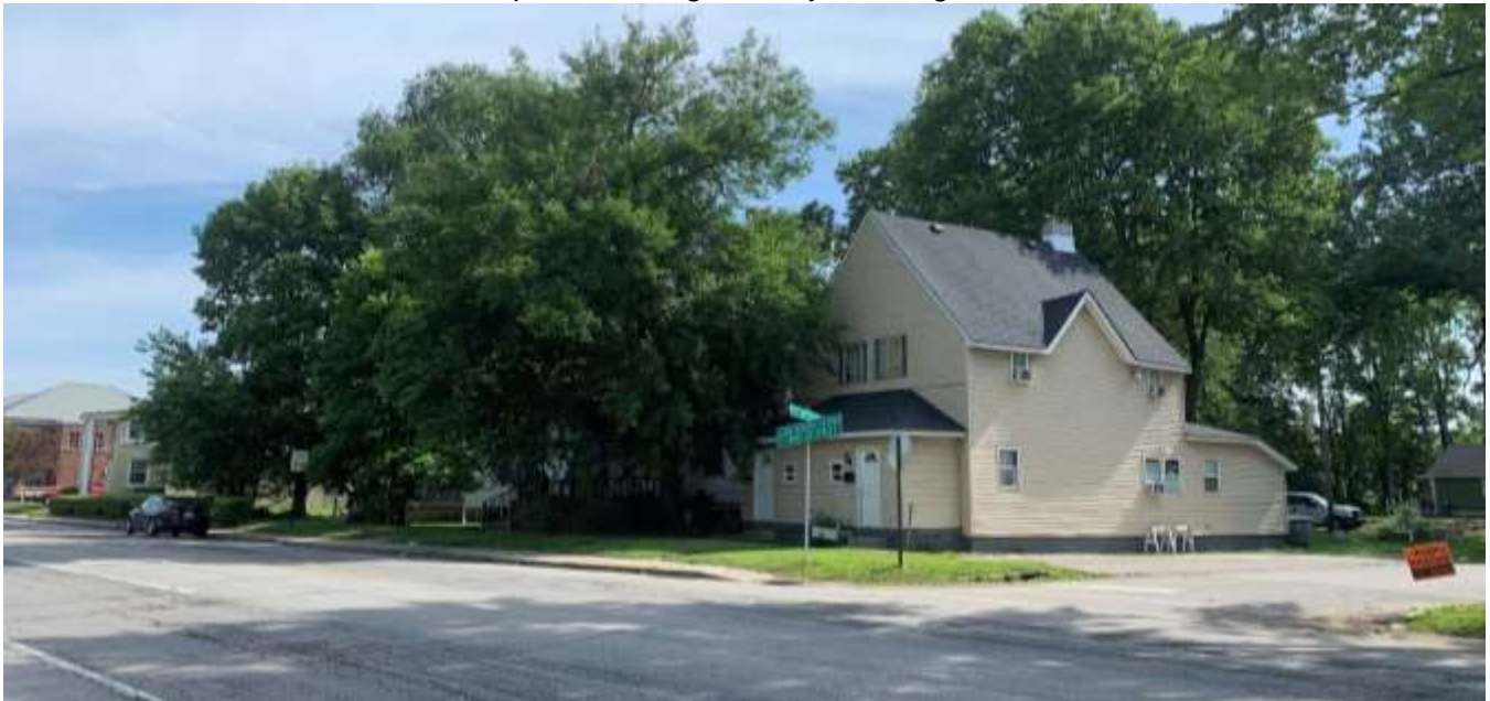
Photo of the duplexes north of the site.
