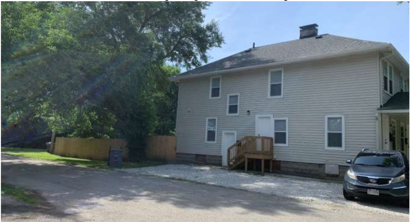
Photo of the north building façade of the existing duplex.
