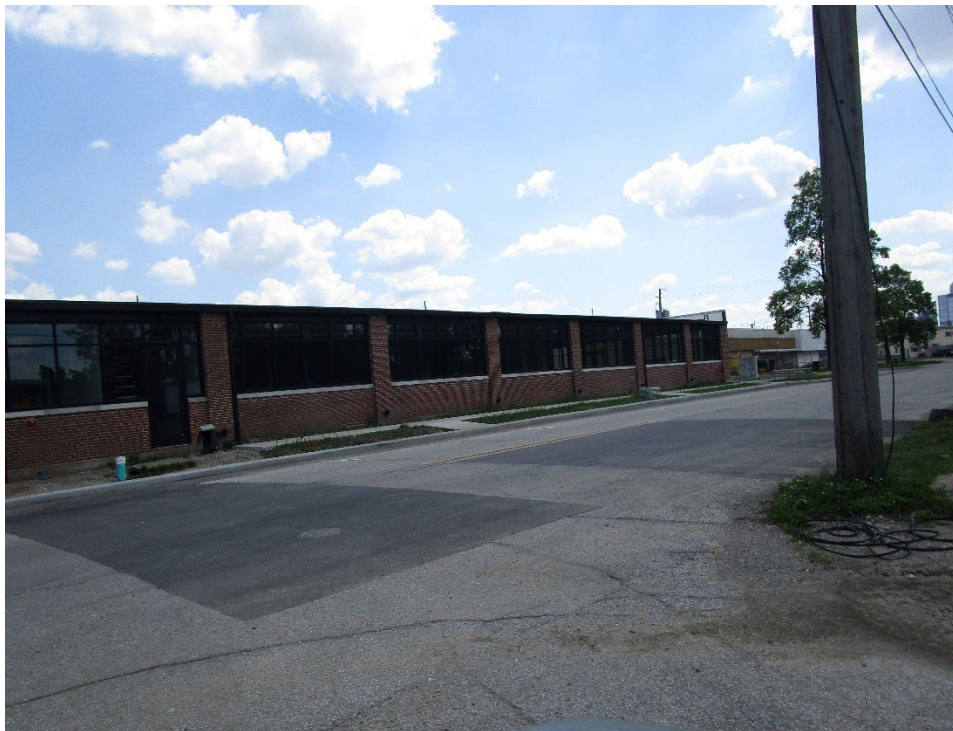
View of site looking southwest across Roosevelt Avenue
