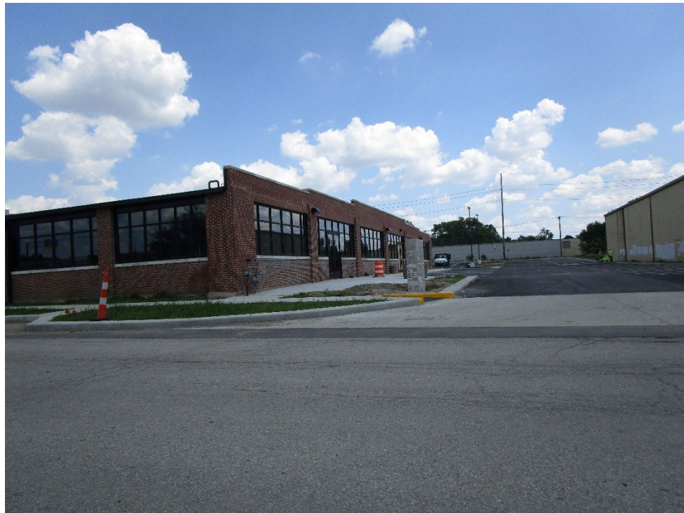
View of western portion of site looking south across Roosevelt Avenue
