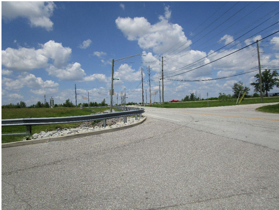
View looking northwest across intersection of Belfast Drive and Flynn Road
