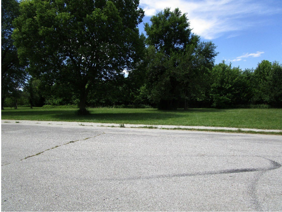
View of site looking north
