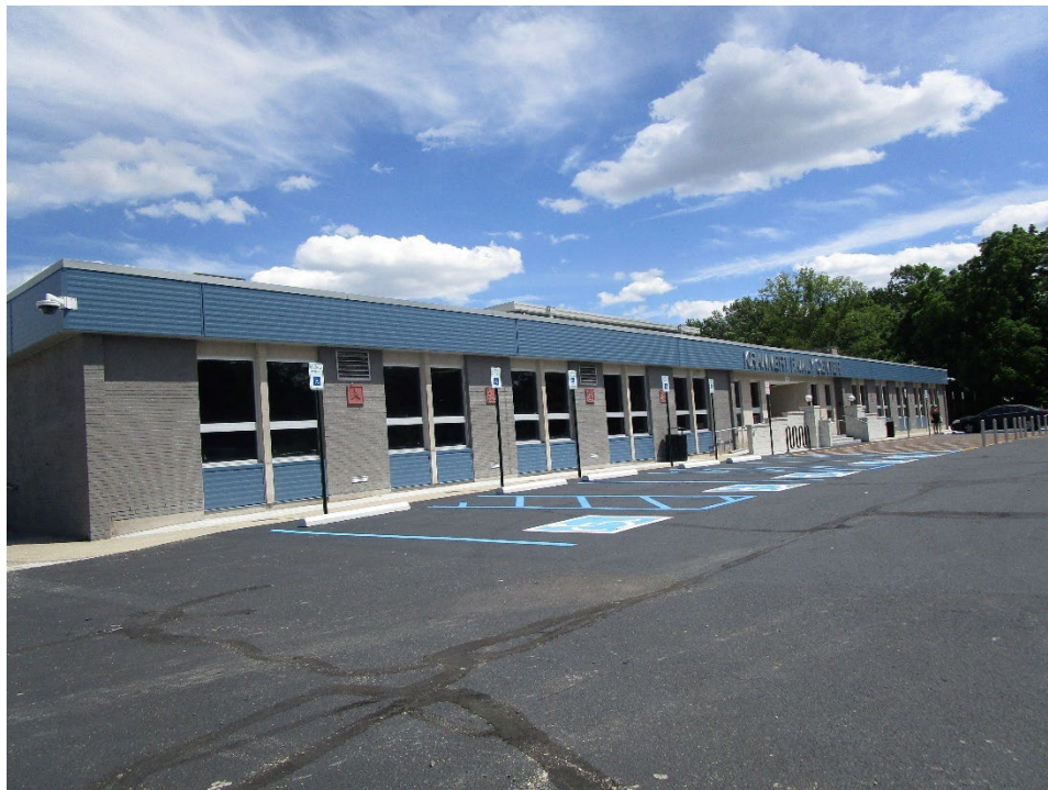
View of community building looking southeast
