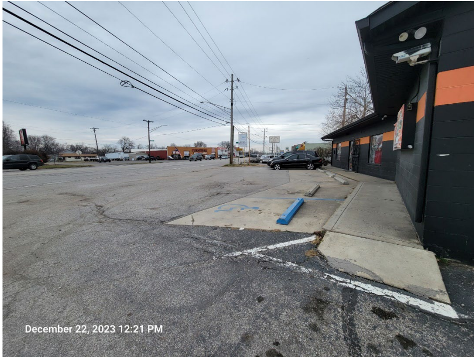
Figure 3 - Subject site looking northeast
