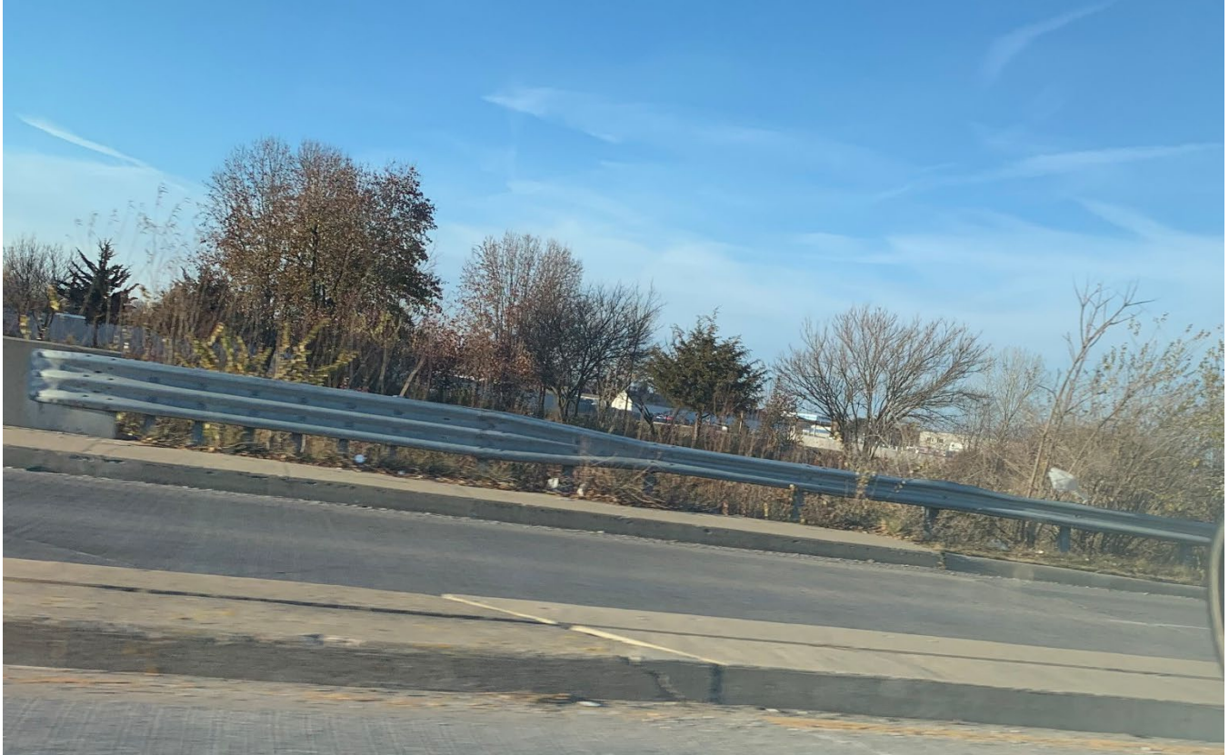
Lot Two Pike Plaza Road frontage, looking north
