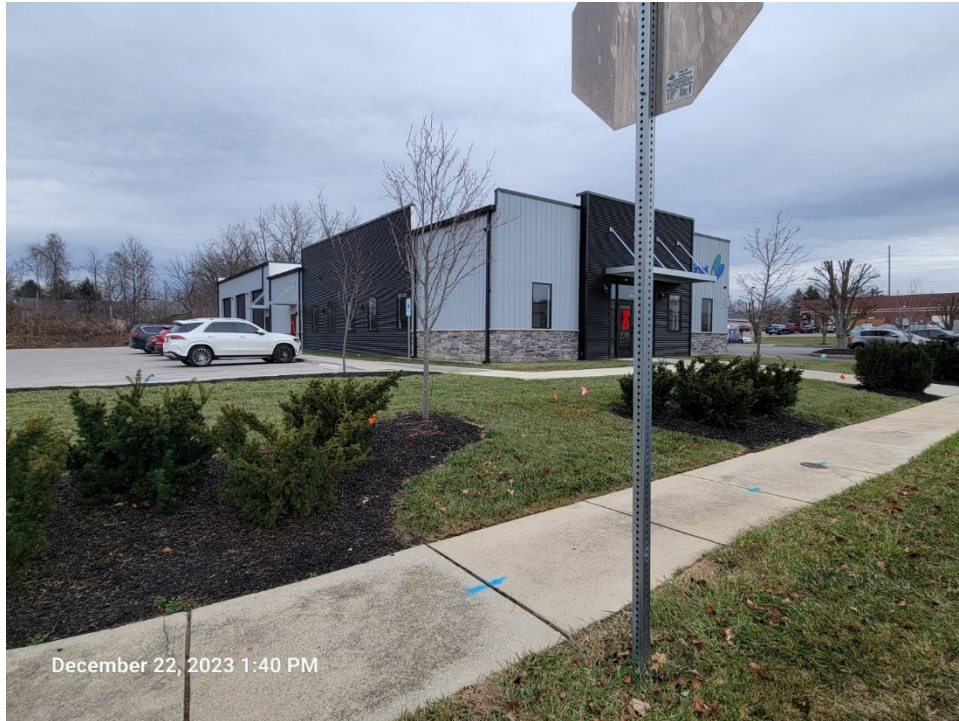
Figure 4 - Existing building on proposed Lot 6B
