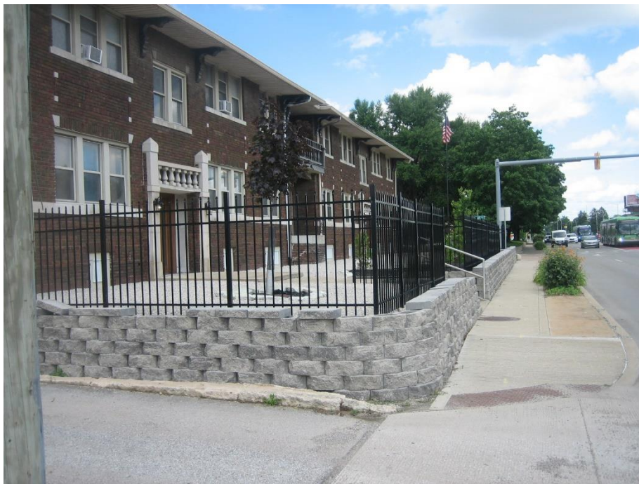
Subject site, 546 East 38 th Street with existing proposed fence height on top of retaining wall, looking east.
