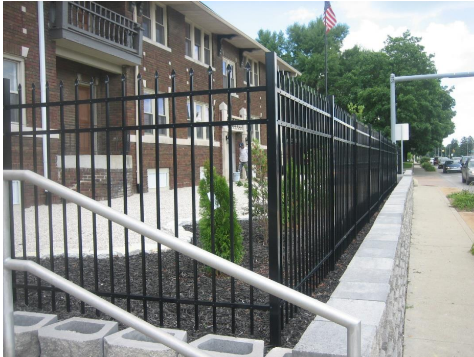
Subject site, 546 East 38 th Street, close-up of existing proposed fence height on top of retaining wall, looking east.
