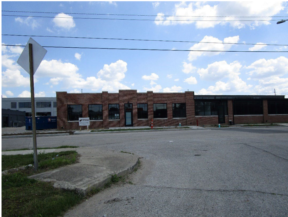
View of site looking south across Roosevelt Avenue
