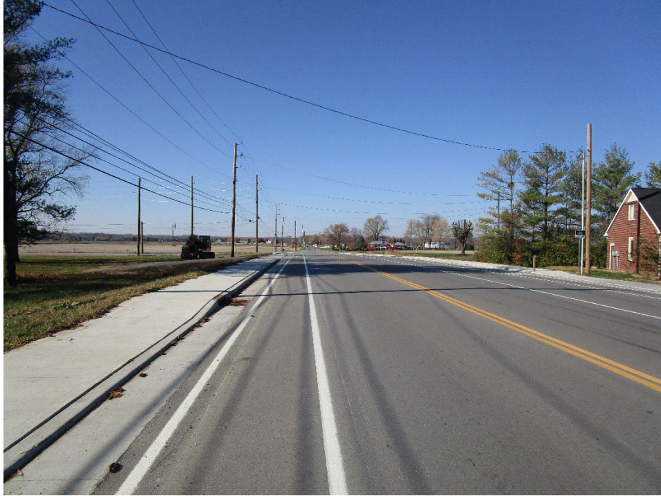
View looking west along Wicker Road
