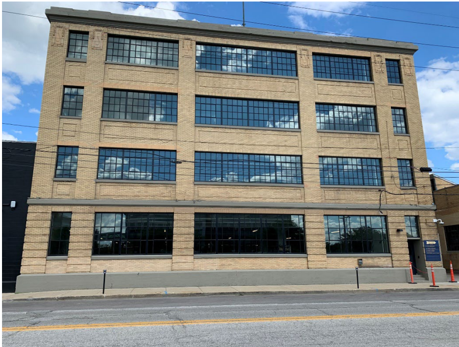
West elevation of subject site – proposed laboratory would be in the first-floor space
