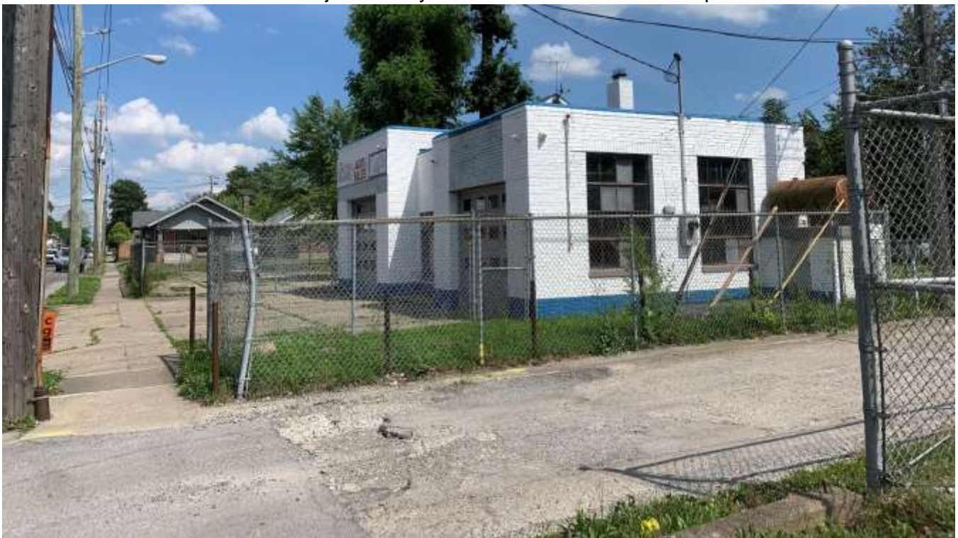
Photo of the subject site looking east.
