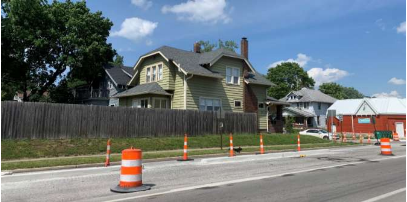
Photo of the residential dwelling north of the site.
